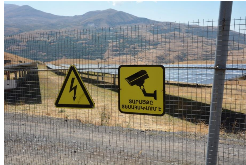
Safety and information signs
