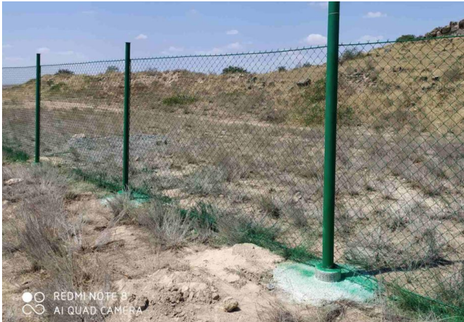
Fencing pole provided with concrete stump
