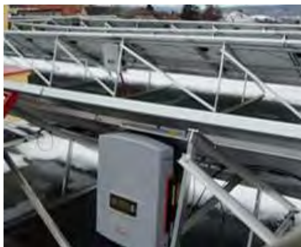
Figure II-30: String inverter mounted under solar PV modules
