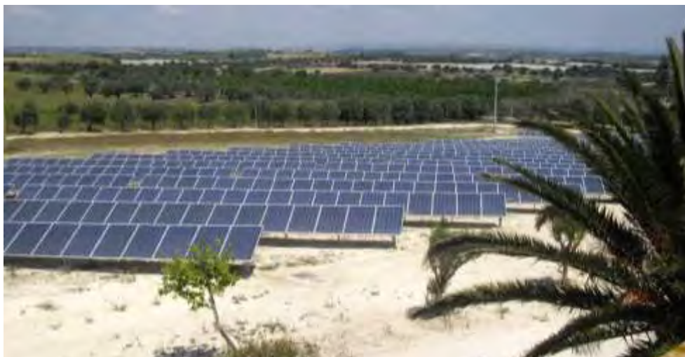
Figure II-24: Example of a fixed mounting solar PV power plant
