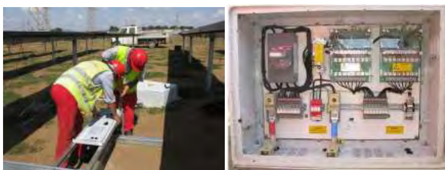
Figure II-46: Electrical routing of cables and installation of electrical boxes
