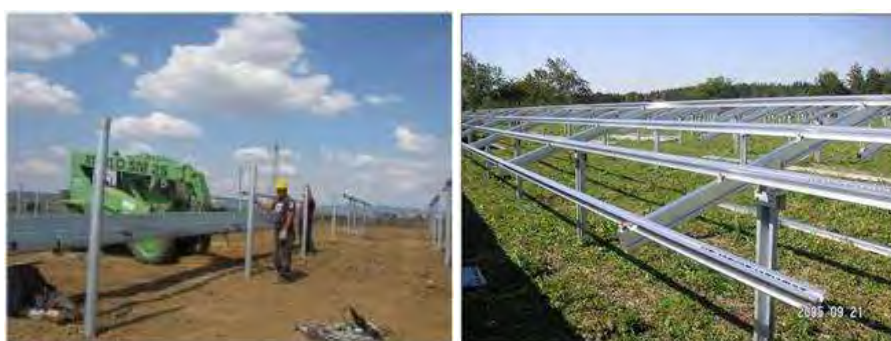
Figure II-45: Examples of mechanical installation of solar PV power plants
